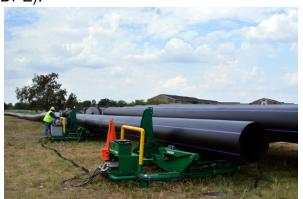
ISCO completed the emergency water reuse pipeline in fewer than four months while the city faced Stage Four drought conditions. The pipeline takes purified water, created from the 7 to 10 million gallons of treated wastewater that is normally released into the Wichita River every day, and after extensive filtration and treatment, supplies it to the public for use.
